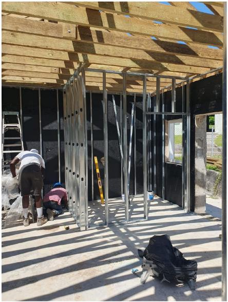
Bitumen applied to the interior walls of Phase 1 for waterproofing (vapor barrier) to combat mold. The same to be executed o Phase II
