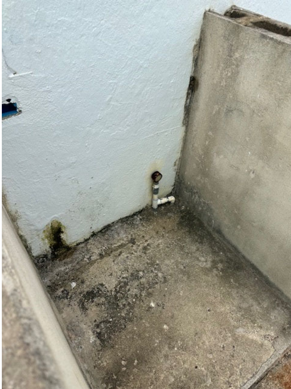
Water Heater Niche
