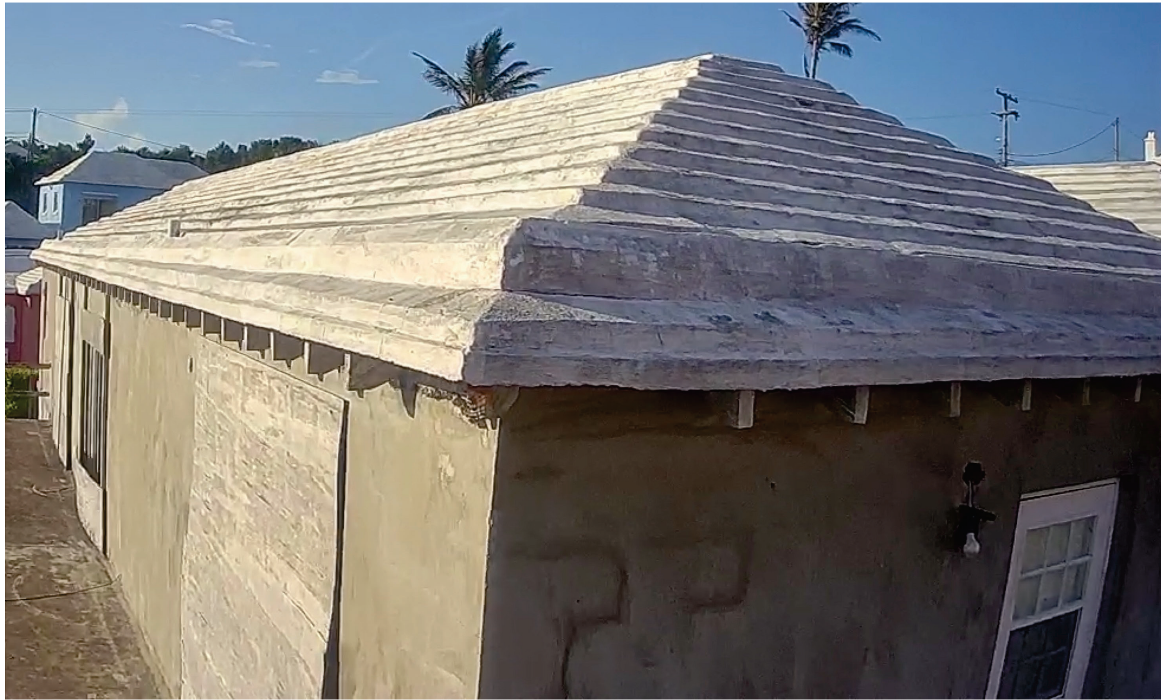
I.1 A0.02 SOUTH EAST DRONE IMAGE ROOF INVESTIGATION
